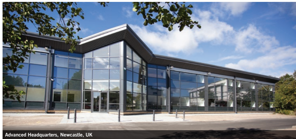
Advanced Headquarters, Newcastle, UK
