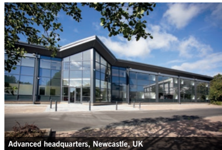
Advanced headquarters, Newcastle, UK
