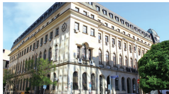
Bulgaria's Communications Regulation Commission Bulgaria's Communications Regulation Commission in Sofia is protected by an Axis EN fire system including false alarm management.
