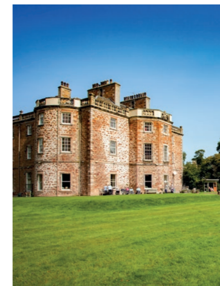
Leuchie House in East Lothian, Scotland, is a respite centre for people with multiple sclerosis. It is protected by an Advanced 4-loop MxPro 5 panel with AlarmCalm false alarm management.
