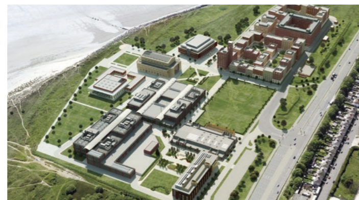
The Bay Campus at Swansea University The Bay Campus at Swansea University is protected by a network of Advanced MxPro 5 fire panels including false alarm management.
