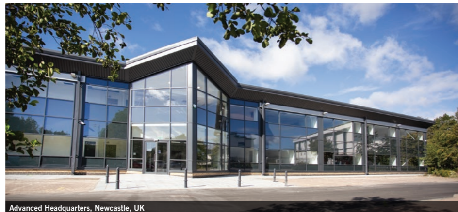
Advanced Headquarters, Newcastle, UK
