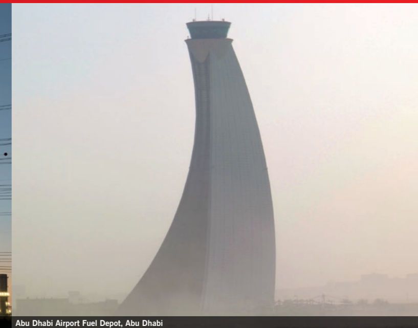
Abu Dhabi Airport Fuel Depot, Abu Dhabi
