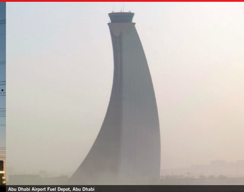
Abu Dhabi Airport Fuel Depot, Abu Dhabi
