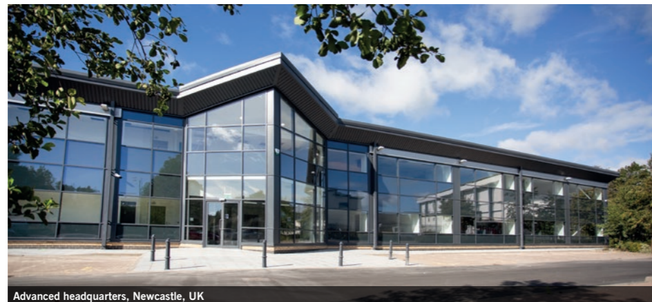
Advanced headquarters, Newcastle, UK
