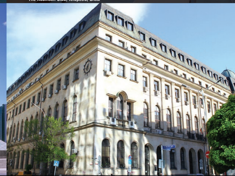
Communications Regulation Commission office, Sofia, Bulgaria
