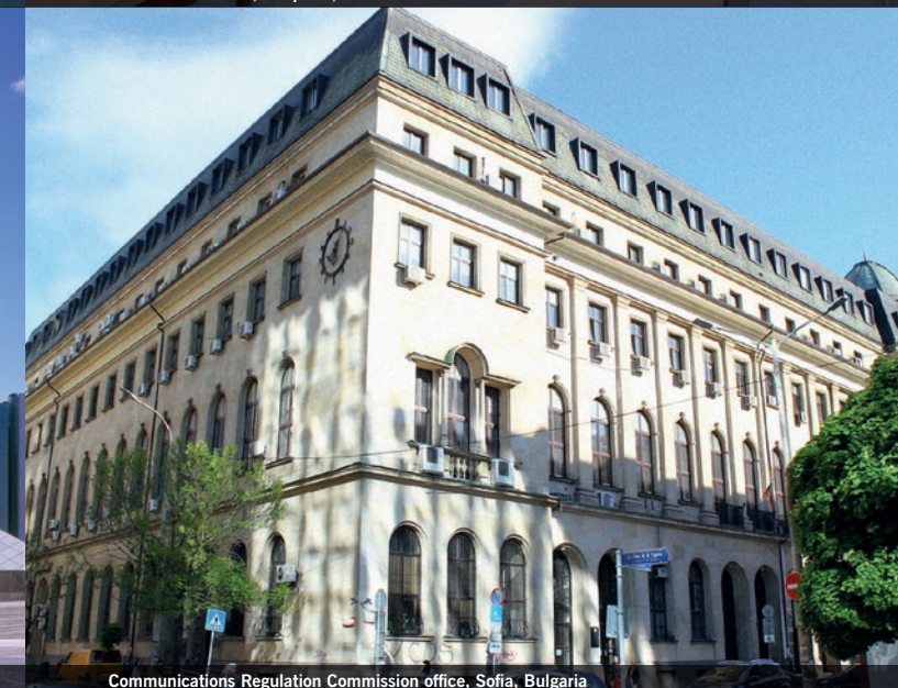
Communications Regulation Commission office, Sofia, Bulgaria
