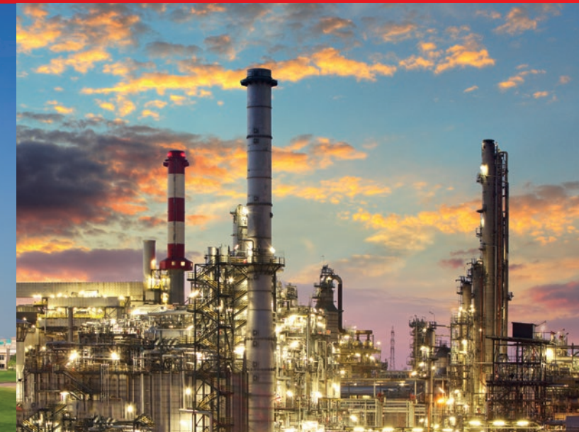
Petronas Refinery, Kuala Lumpur, Malaysia
