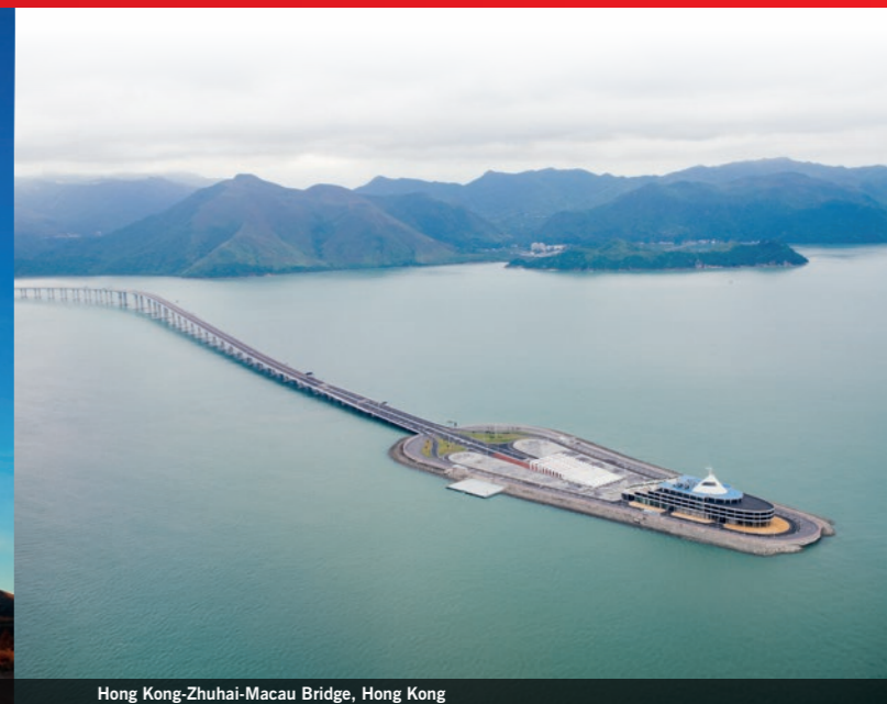
Hong Kong-Zhuhai-Macau Bridge, Hong Kong
