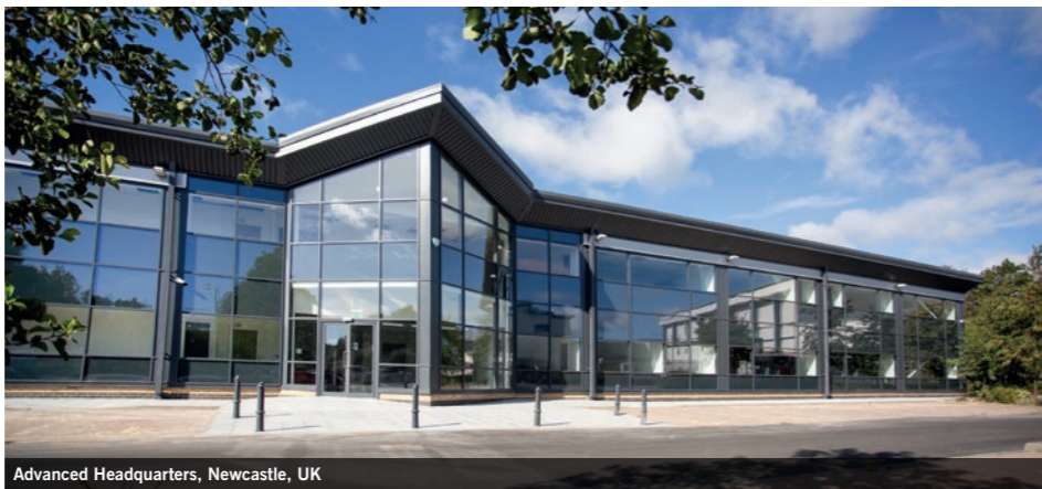
Advanced Headquarters, Newcastle, UK
